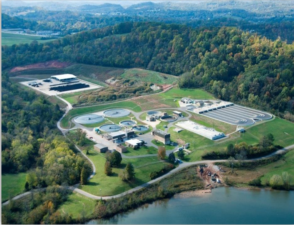
Aerial View-Notice Class “A” Composting Facility in Background Maryville Regional Wastewater Treatment Plant Maryville, Tennessee
