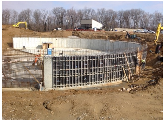
Pictured above is construction of the 160 ft. diameter Clarifier North Wastewater Treatment Plant Henderson, Kentucky
