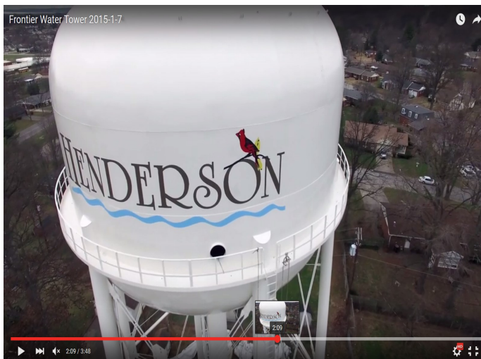
Frontier Water Storage Tank Flyover Compliments of HWU Staff Member Henderson, Kentucky
